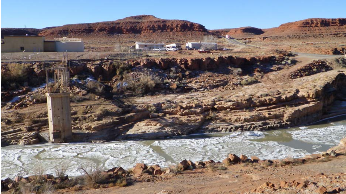
Figure 5-4. View looking across the river channel to the existing intake structure (Photo December 2013).
