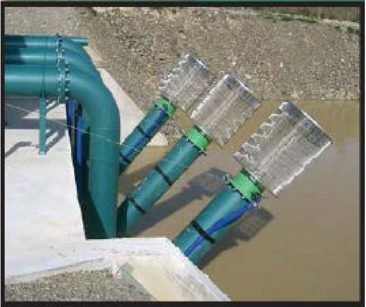
Figure 5-15. Typical Self Cleaning Screen Installation.
