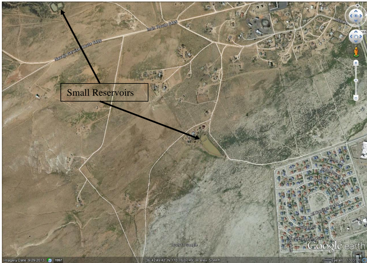
Figure 4-2. View of Small Dams built on secondary drainage adjacent to Kayenta, Arizona.
