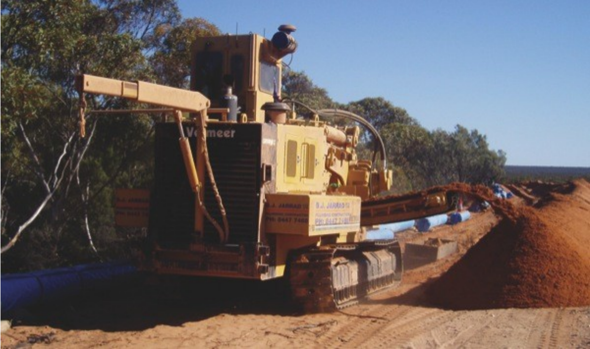
Figure 6-12 – Typical Trenching Machine – Source PipelinesInternational.com
