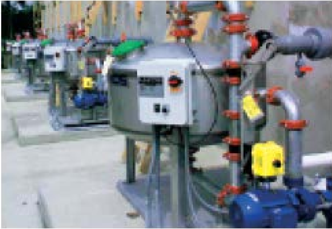
Figure 5-19. Multiple Sand Filter Installation(Lakos).
