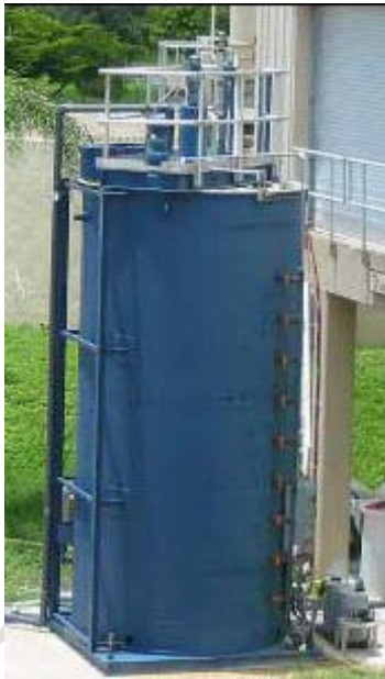
Figure 7-6. Packaged Clarifier(Siemens Water Technologies).
