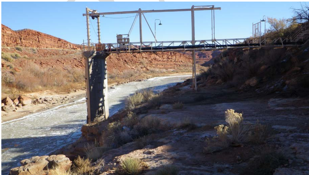
Figure 5-3. View looking upstream at the existing water treatment plant intake structure(Photo December 2013).
