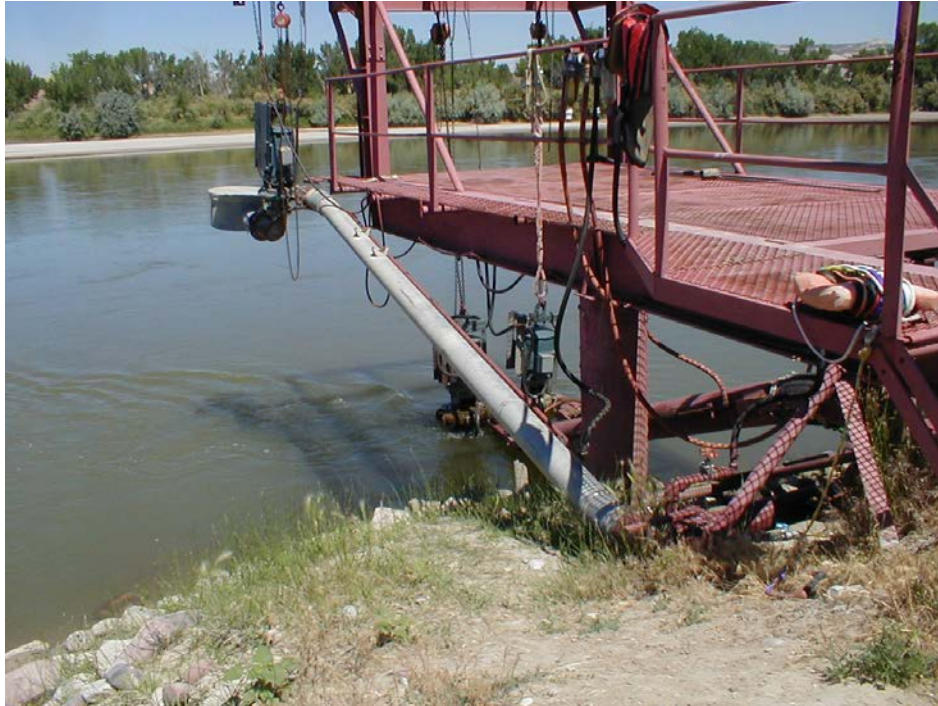
Figure 5-9. Example of a suspended pump intake structure.
