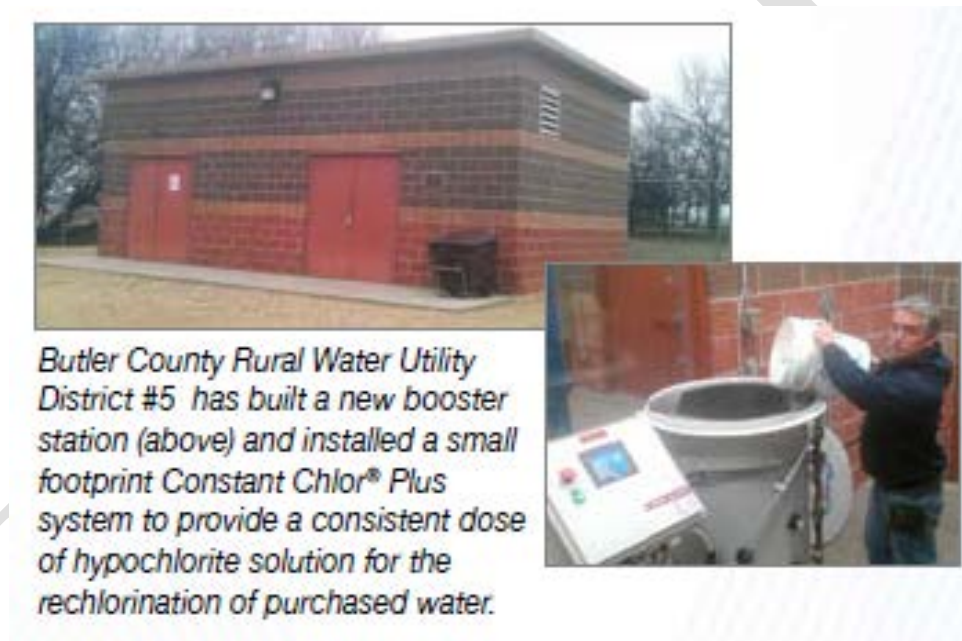
Figure 7-9. Chlorine Booster Station. Source Arch Constant Chlor®
